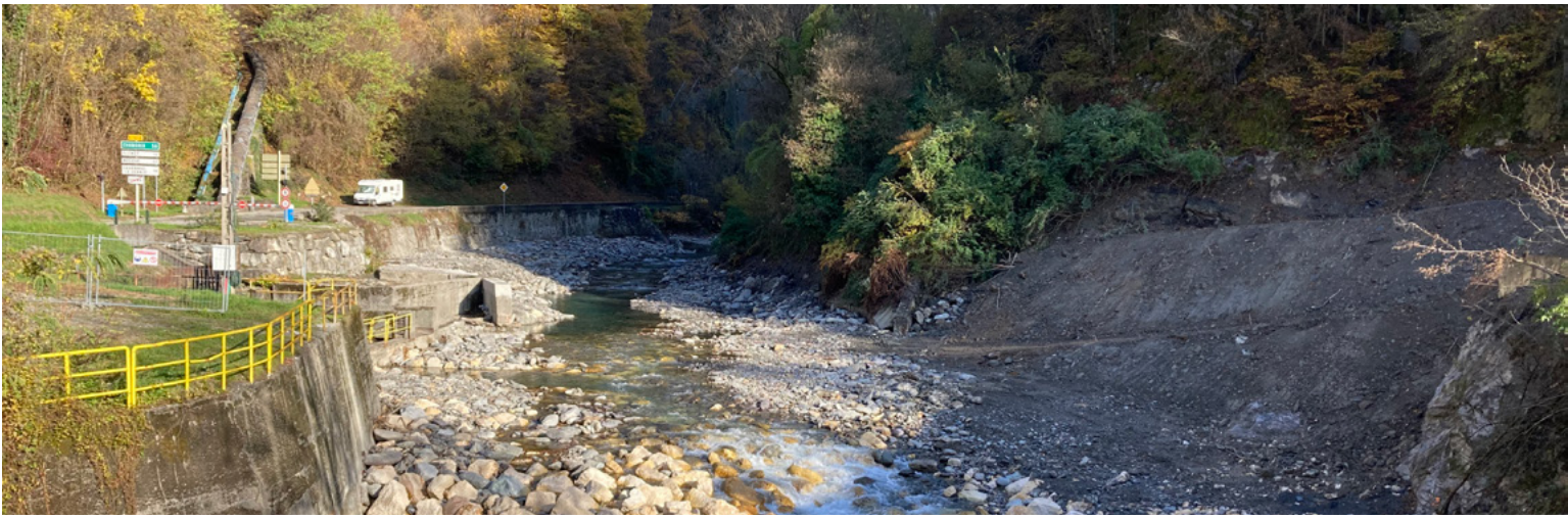
New ramp at the Mollières weir
