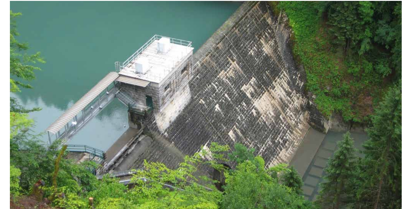
The Mottets dam on the River Arly supplies around 40% of the electricity required by the Ugine site
