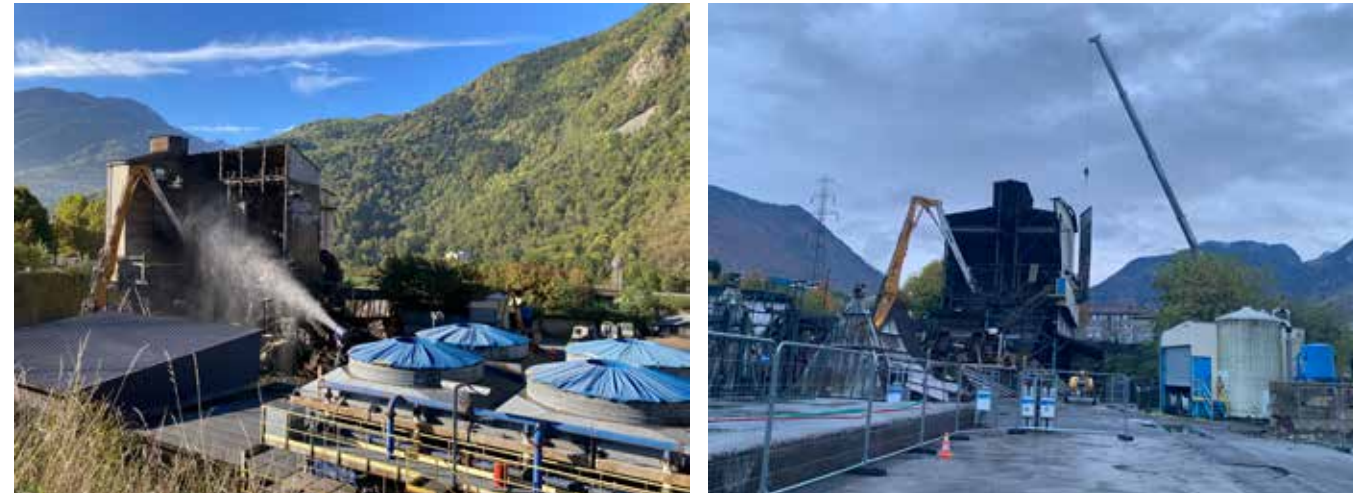
Demolition at the Léchère site
