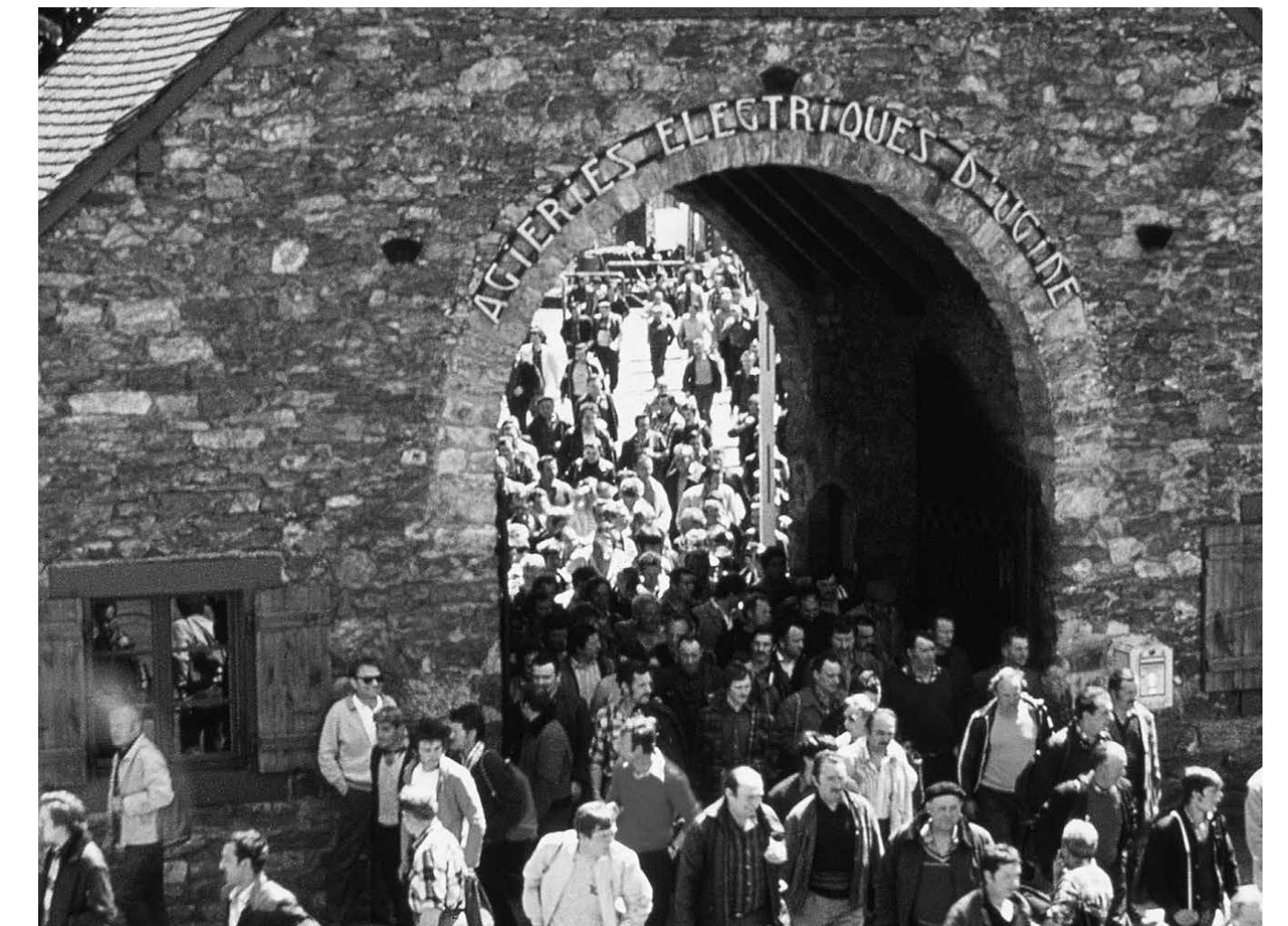
Rolled out of the Ugine Electric Steelworks
